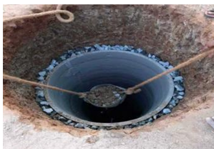
Figure 4: Construction of discharge
